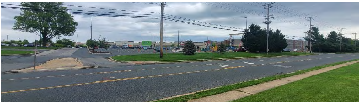
Tollgate Marketplace across Tollgate Road with Dick's construction in foreground
