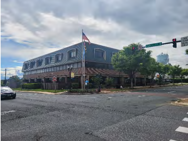
County office building at 220 S. Main St.
